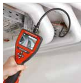
Inspection of hollow spaces
