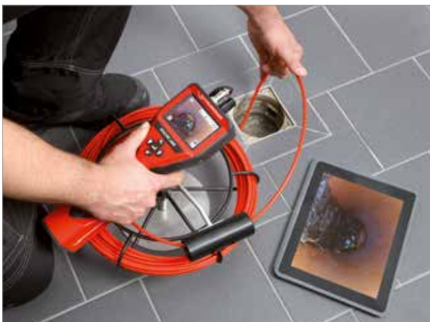
Inspection of basin drains
