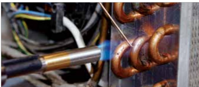
Brazing in refrigeration / air-conditioning technology
