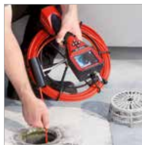
Inspection of rain downpipes
