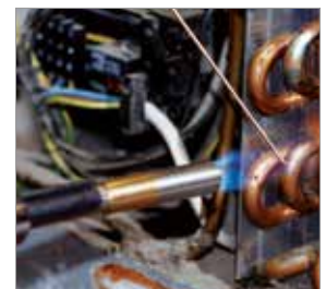
Brazing in refrigeration / air-conditioning technology
