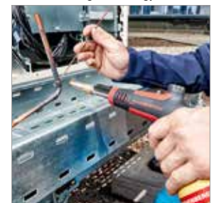
Brazing in refrigeration / air-conditioning technology
