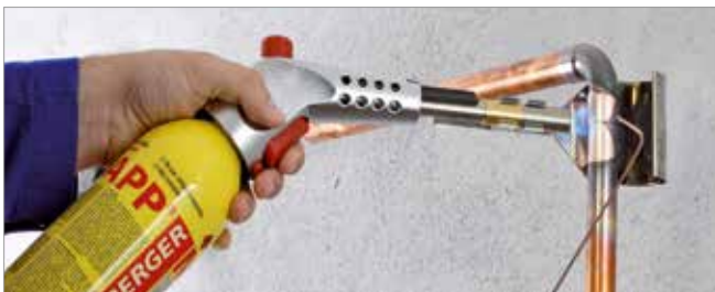
Brazing in gas installation
