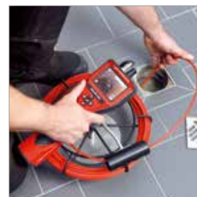
Inspection of floor drains
