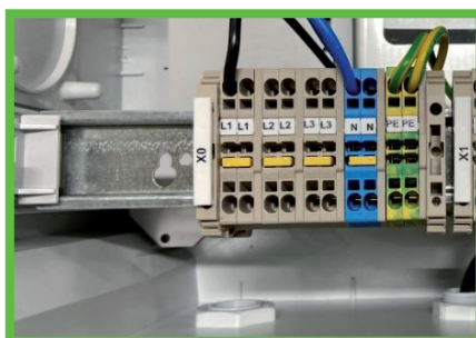
Figure 14 A: 230V connection PURE
