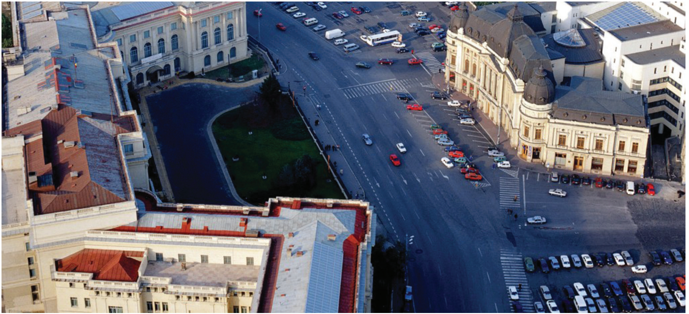
Bucharest, Romania – Multi-family and commercial buildings supplied with district heating.
