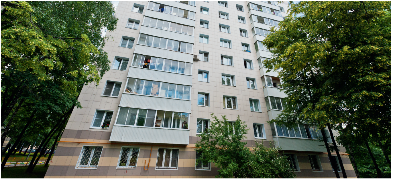
Moscow, Russia – Multi-family buildings with district heating inside.
