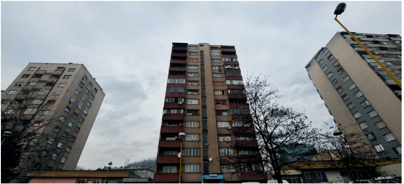
Tuzla, Bosnia & Herzegovina – Multi-family buildings with district heating inside.
