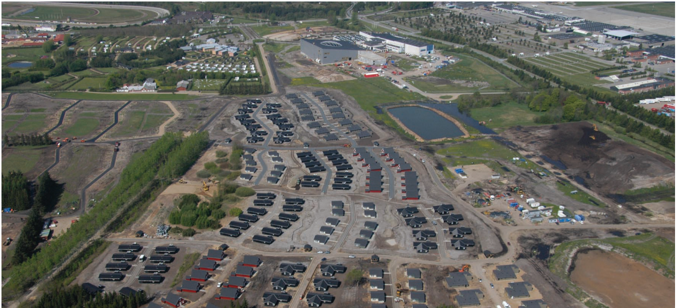
Billund, Denmark – One-family houses supplied with district heating.
