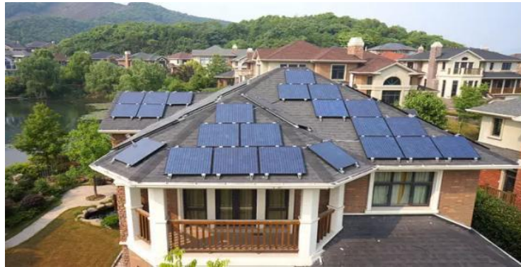
multiple roof orientation
