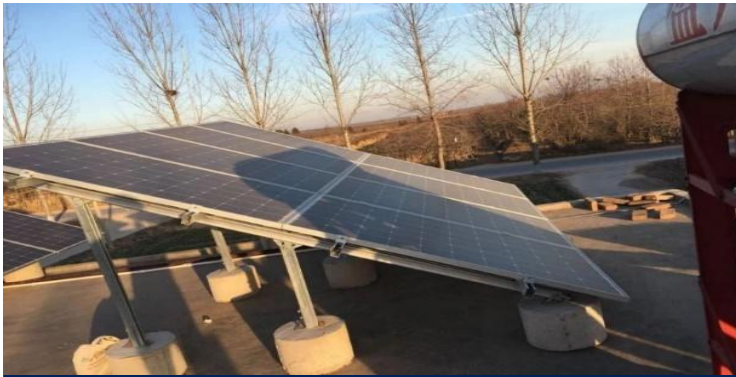
Shielding of equipment
