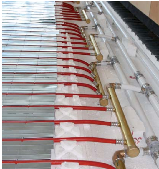
Roth underfloor heating, multi-purpose hall, Dautphetal, Germany
