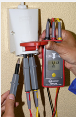
Validate receptacle wiring
