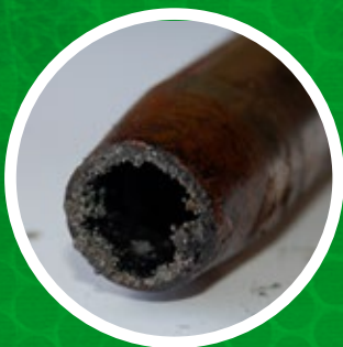
WITHOUT PROTECTION, AFTER WELDING
